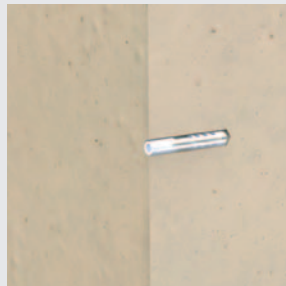
2. Insert suitable dowel
