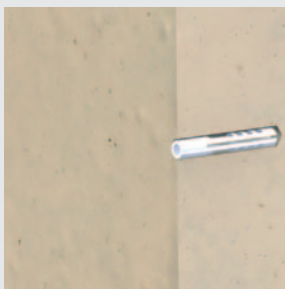
1. Insert suitable dowel
