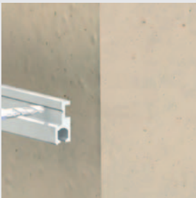
1. Drill hole in track
